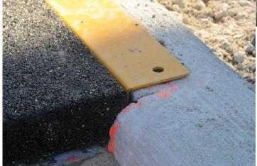
The Threshold System provides long-term support that is independent of the preparation of the base materials at the edge of the playground. The **EVERPLAY** Threshold is ADA compliant and provides for no change in vertical height greater than 1/4" and the sloped edge is at less than 1:2 and less than 1/4" in vertical height.
