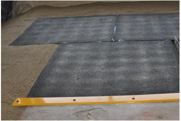
The EVERPLAY PlayMats54 are manufactured in 5' x 4' x 2" size to ensure compliance with the minimum width for the ADA Accessible Route. Placing these in combination will ensure the maintenance of the require Accessible Route.
